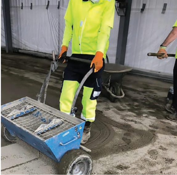
Hatcrete dry-shake – hopper application. (Photo: Nationwide Concreting Ltd.)
