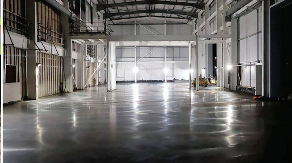
Hatcrete dry-shake with cure and seal. (Photo: SJ Stanbury & Sons Ltd.)
