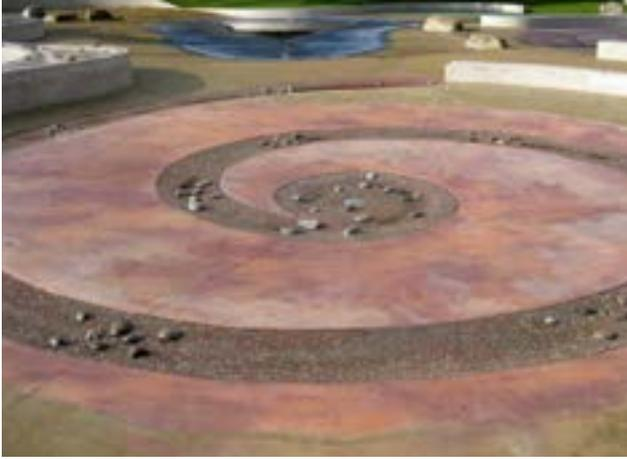
**Figure 2:** A project using seeded, integral colour, pink dry shake, which was shot blasted.
